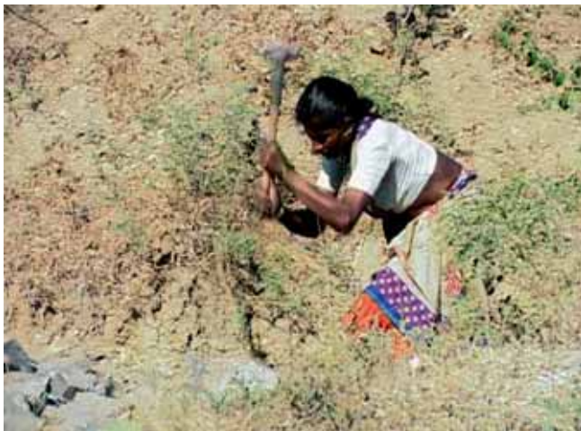
Wells are dry for six months a year in this woman's village; she and fellow villagers have to migrate and work in road building
