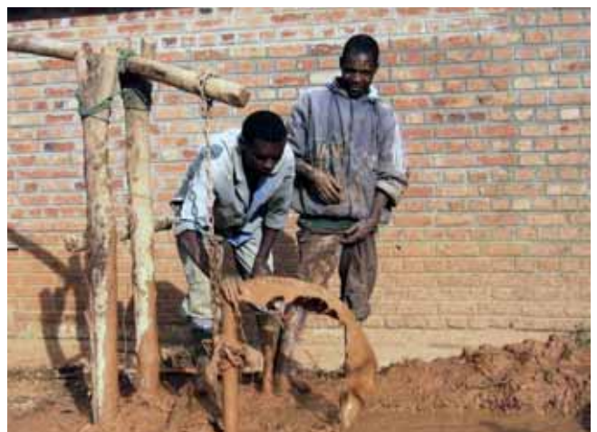
Well drilling is an important cost factor in irrigation; the cheap 'rota sludge method' of drilling developed in Latin America is now being spread in Africa
