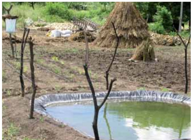
Low-cost water storage bag and tank made of plastic sheeting developed in India, costing around US$ 80 for 10,000 litres
