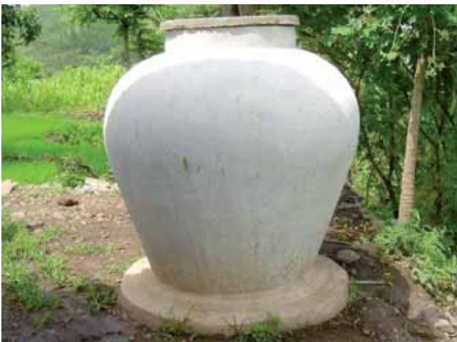
Modified Thai jar tank of 3,000 litres developed in Nepal
